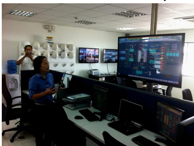
Ms. Rowena Dalosa, Rowena Dalosa, Plant Manager, East La Mesa Water Treatment Plant, Water Supply Operations. She is explaining the automated system of at the main operation desk of the water purification process (coagulation/flocculation, sedimentation, filtration and disinfection).
